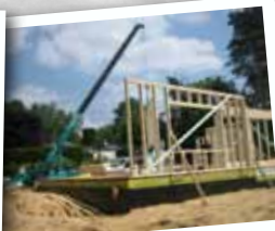
Timber Frame Work
