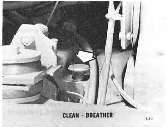
Figure 186 TRANSMISSION & CONVERTER BREATHER
