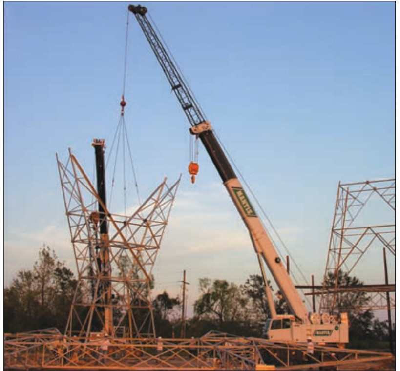
Full power telescopic boom with extension installed. Quickly adjust crane boom configuration during assembly of structures of varying heights.
