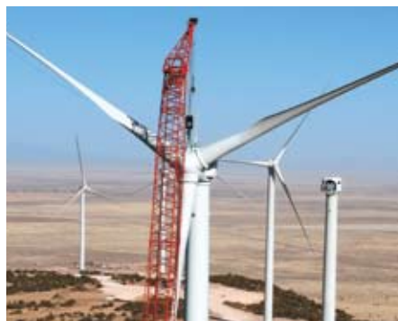
Lattice-boom crawler cranes
