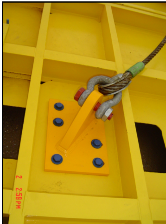
Figure 19 - Lifting Pad Eye and Sling Connection
