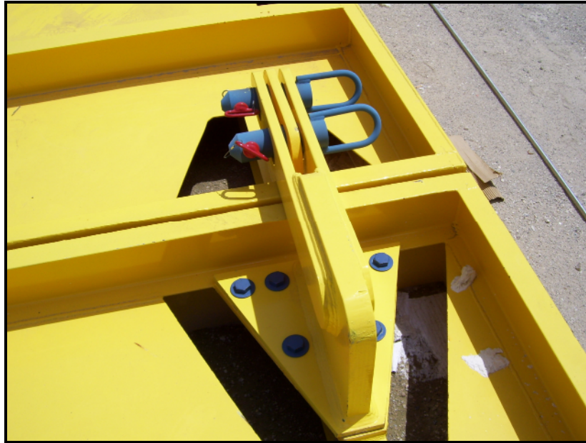
Figure 17 - Bolted and Pinned Hinge Connection
