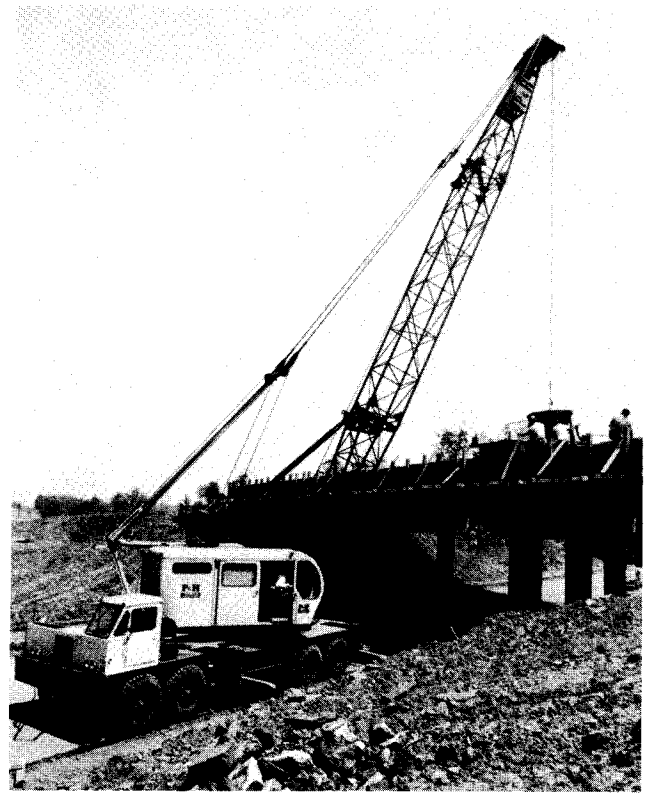
High-production concrete pouring is made to order for Magnetorque® swingers — fast and smooth cycling with never an adjustment.
