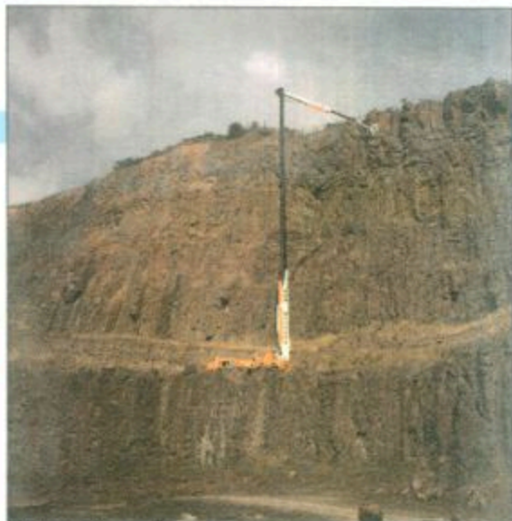
Safety survey of quarry face.
