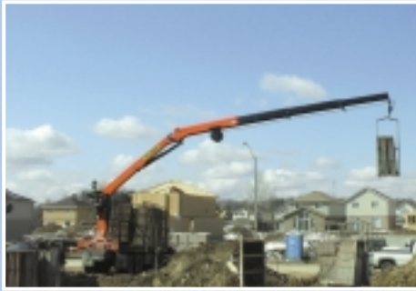
Up to 60' horizontal reach for today's hard to access job sites
